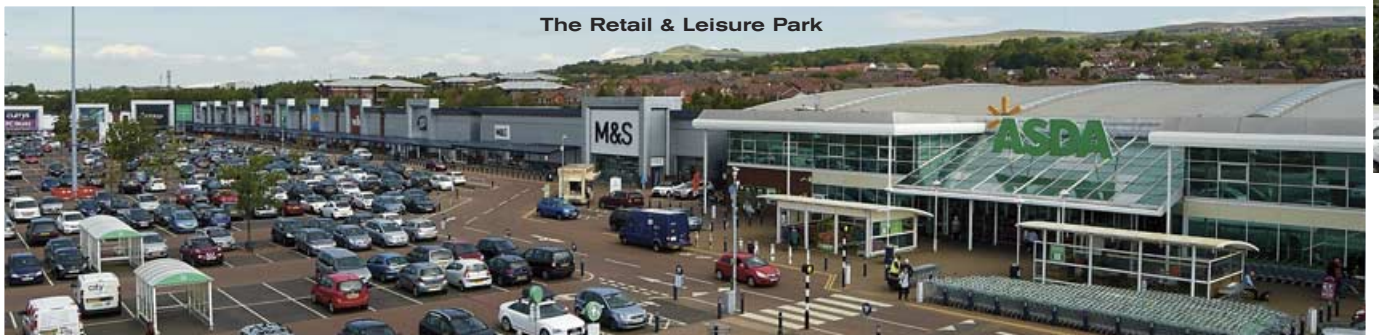
Parklands 5A / 5B & Multi-Storey Car Park Middlebrook
